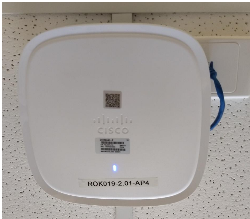
Figure 2.4.2.2 - Method 2 Suitable where solid ceilings are used.
