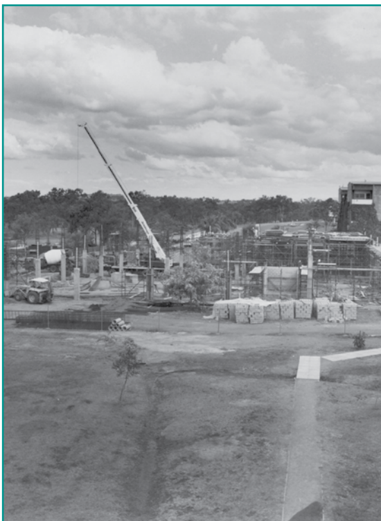
Construction of the Library building
